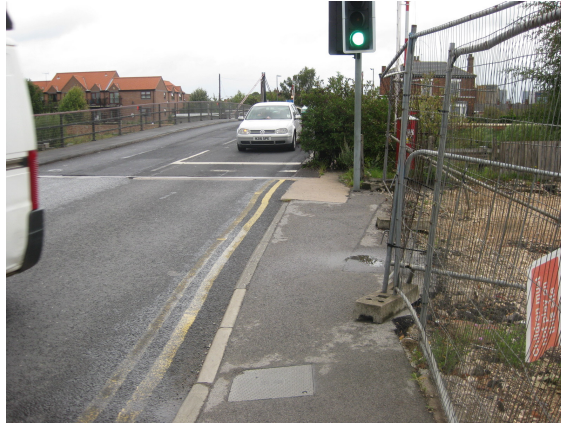
Photograph 1 – existing footway provision on PFS Frontage
